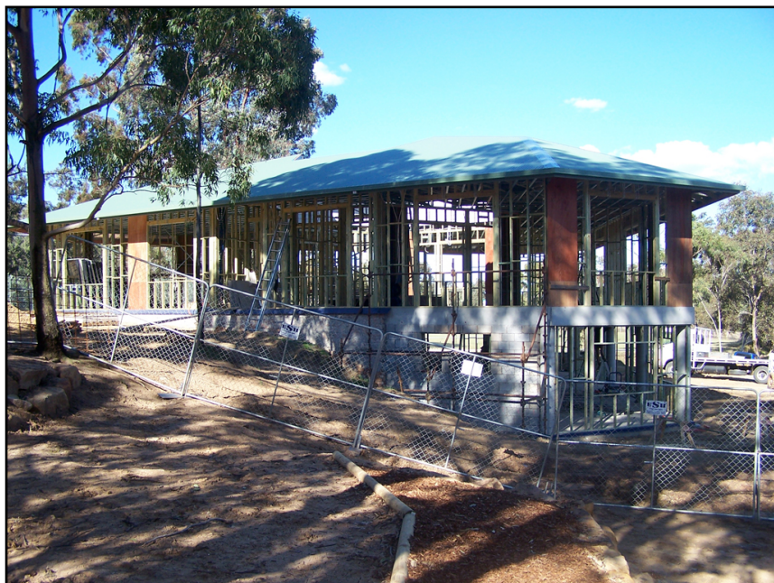
Building 7 under construction.
